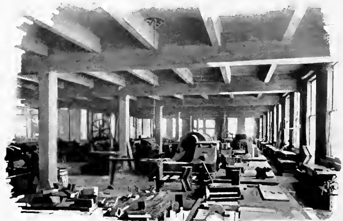
General View on First Floor of Pattern Department
